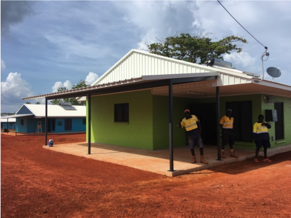
New house under construction, Galiwin'ku, Northern Territory
