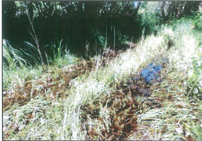
Figure 4 - Sporadic inundation of the track from ground surface water moving south (from right to left) toward Clybucca Creek.
